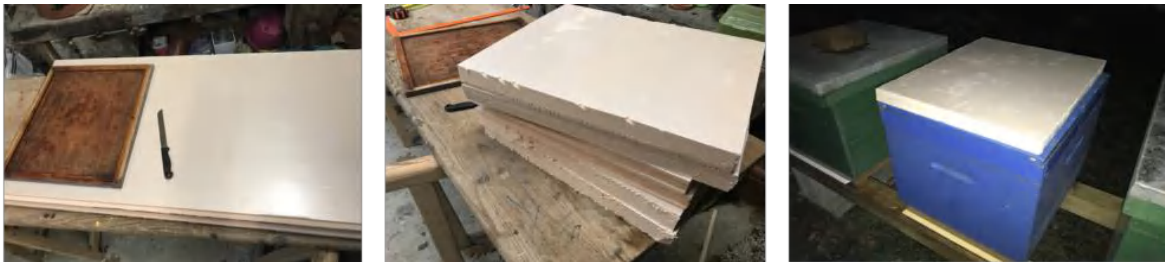
Cutting of 40mm polystyrene boards and installation between the roof and the feeder.
