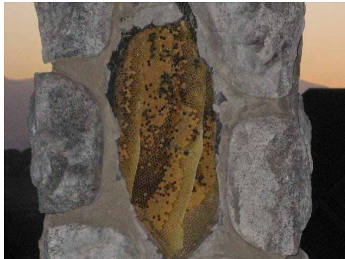
Figure out how to remove the bees in a way that can be easily repaired when done.
