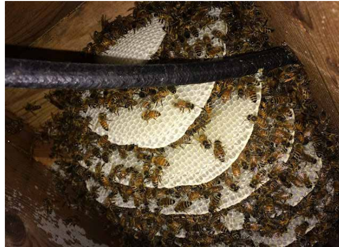
Cavity with honey bees and electrical supply line poses risk of death if improperly removed.
