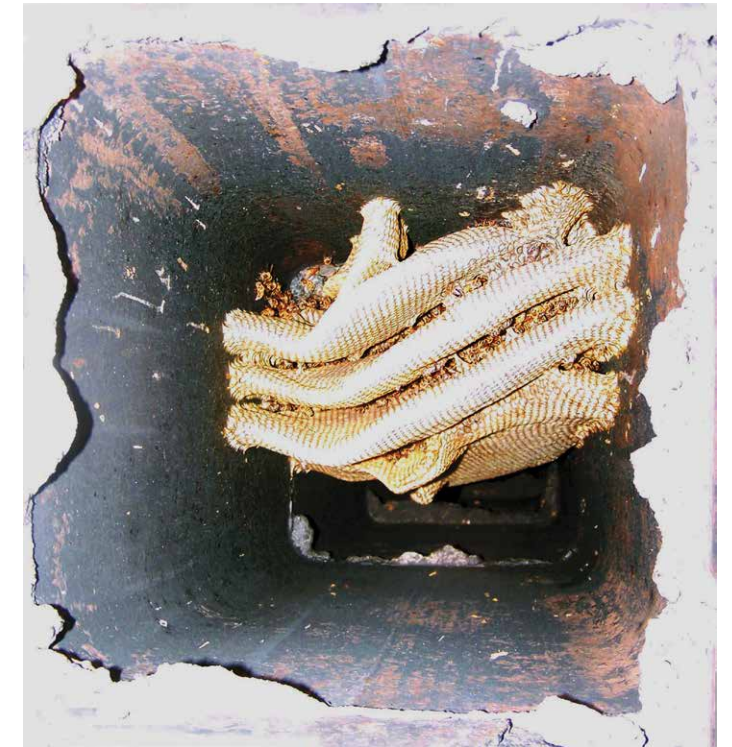
Chimney removals are the most difficult, but with the right know-how it is possible.
